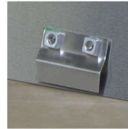
Completed bracket inside Growhouse
