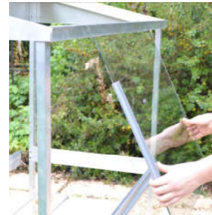
C. Fitting the glass
