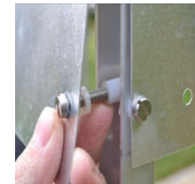
Nylon spacers on infill plate
