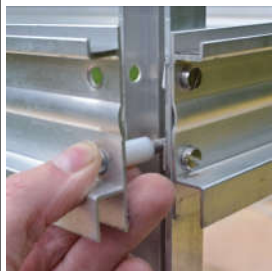
Nylon spacers on bolt
