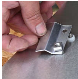
White spacers on infill plate
