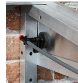
Inlet and link pipe
