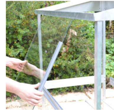
A. Fitting the glass
