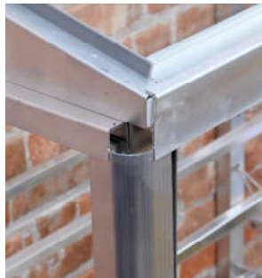
Corner trim in place
