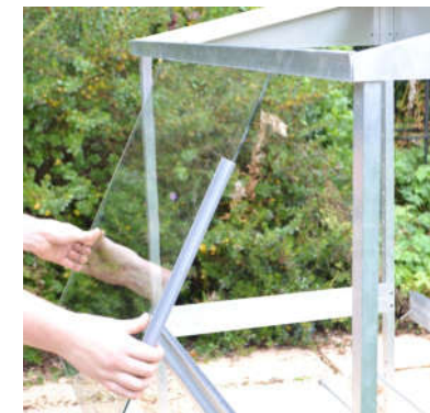
A. Fitting the glass
