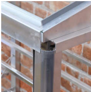
Corner trim in place
