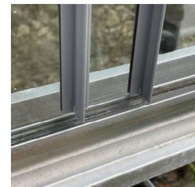
Glass in channel with two sheets overlapping
