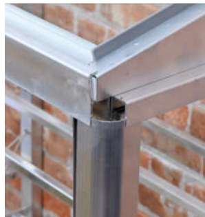
Corner trim in place
