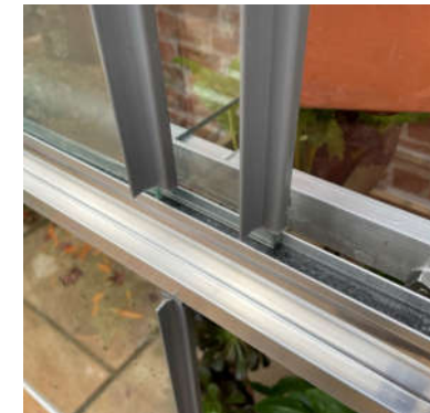
Glass in channel with two sheets overlapping
