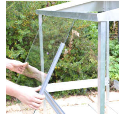
A. Fitting the glass
