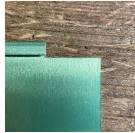
Notched edge of first infill plate on BX5 & CX5
