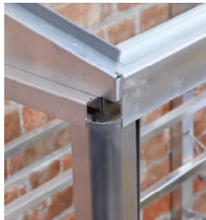
Corner trim in place
