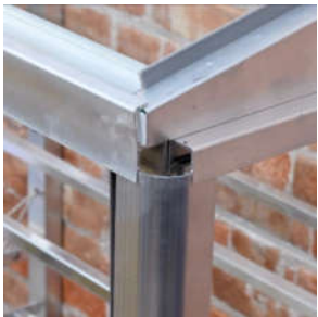
Corner trim in place
