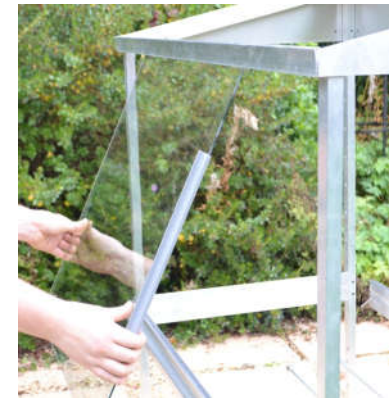
A. Fitting the glass
