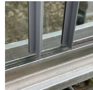
Glass in channel with two sheets overlapping
