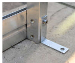
ANCHORAGE BRACKET FITTED
