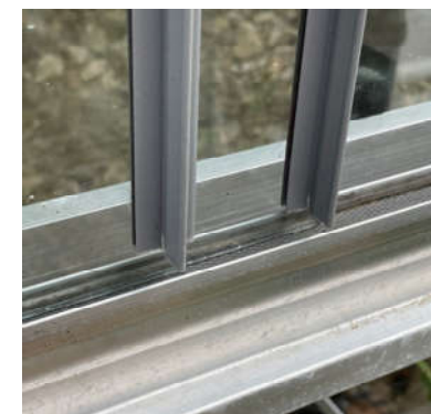
Glass in channel with two sheets overlapping
