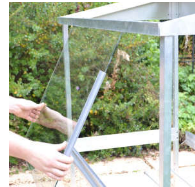
A. Fitting the glass
