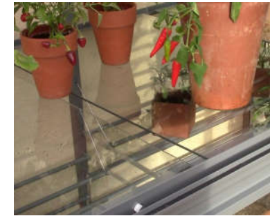
D. Centre staging fitted
