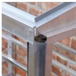
Corner trim in place
