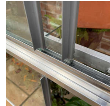
Glass in channel with two sheets overlapping
