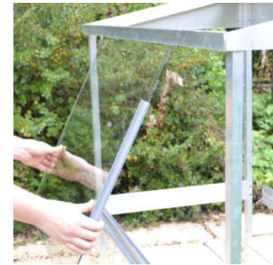
A. Fitting the glass
