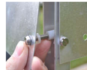
White spacers on infill plate
