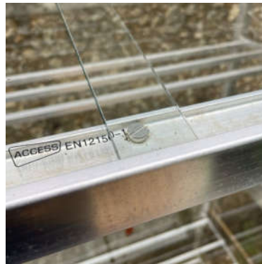
Roof glass overlapping
