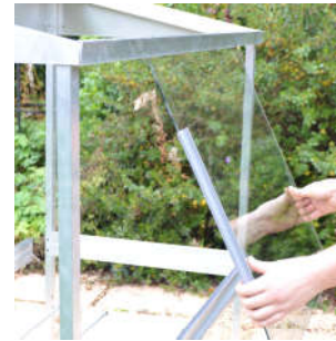
C. Fitting the glass
