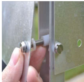
Spacers on infill plate
