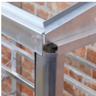
Corner trim in place
