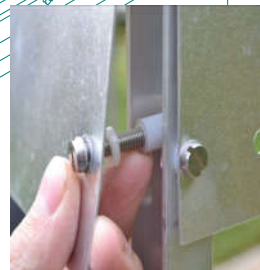
White spacers on infill plate
