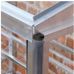
Corner trim in place
