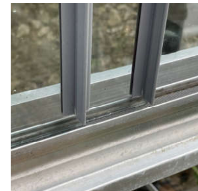
Glass in channel with two sheets overlapping
