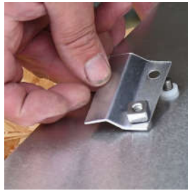
Nylon spacers on infill plate
