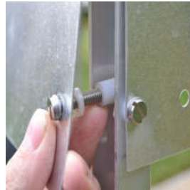
Nylon spacers on infill plate
