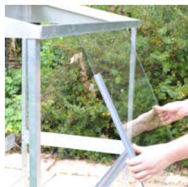
C. Fitting the glass
