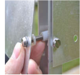
Nylon spacers on infill plate
