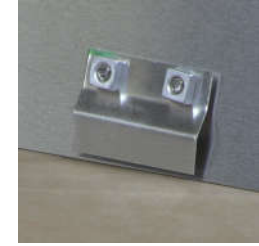
Completed bracket inside Growhouse
