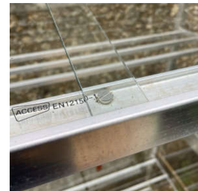
Roof glass overlapping
