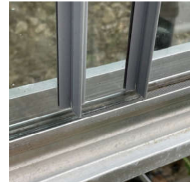
Glass in channel with two sheets overlapping
