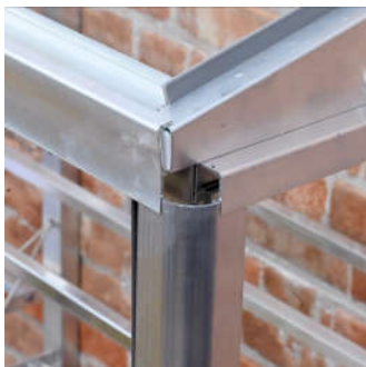
Corner trim in place
