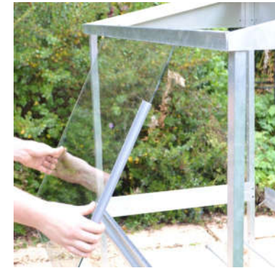
A. Fitting the glass
