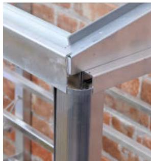
Corner trim in place
