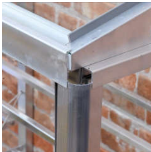
Corner trim in place
