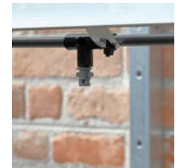
Nozzle strapped to 'L' bracket
