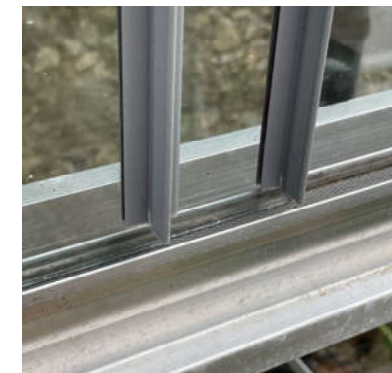
Glass in channel with two sheets overlapping
