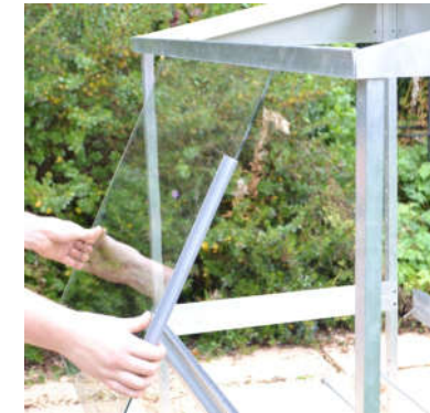
A. Fitting the glass
