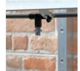
Nozzle strapped to 'L'
