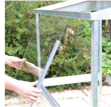
A. Fitting the glass
