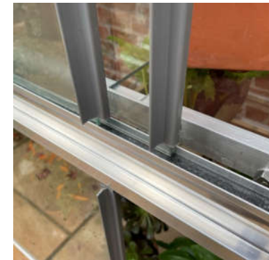
Glass in channel with two sheets overlapping
