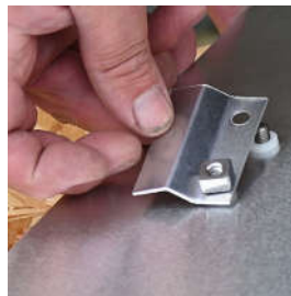
White spacers on infill plate
