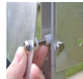
Nylon spacers on infill plate
