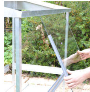
C. Fitting the glass
