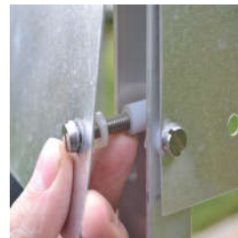
Nylon spacers on infill plate
