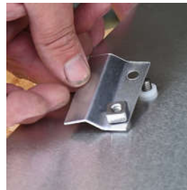
Nylon spacers on infill plate
