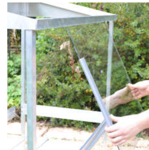
C. Fitting the glass
