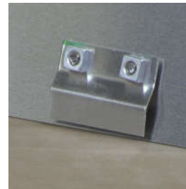
Completed bracket inside Growhouse
